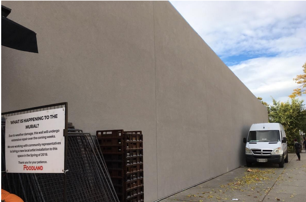
Wall site photo
